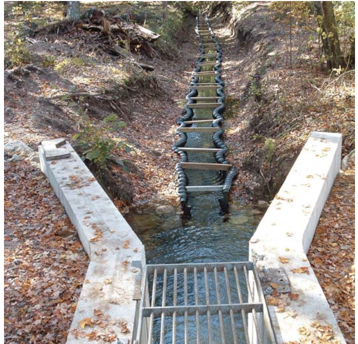
View downstream from Middle Pond herring run ladder showing 140 ft of newly installed FastDitch lining.
