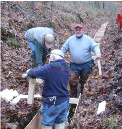
Herring Run flume being relined and braced on a January morning.
